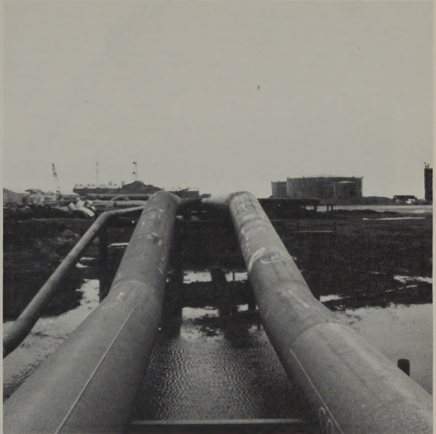
(Above) The pipeline is set on vertical support modules to protect it from permafrost in this inhospitable environment.
